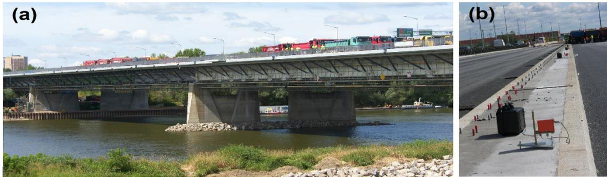
**Figure 2.** Monitoring of the deflection during static bridge load testing; (a) view of the bridge; (b) inclinometers location at the bridge deck.
