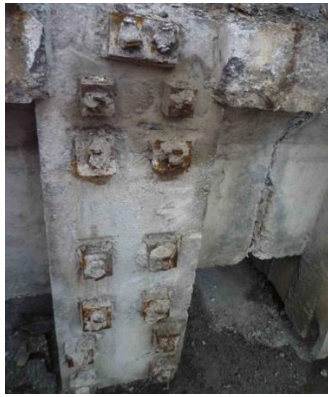
Figure 1a). No sheathing on the anchors – Figure 1b). Crack in the girders - Bridge Podbiel Bridge Nizna
