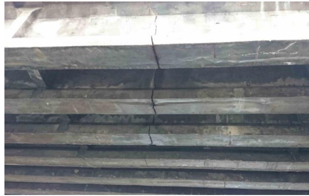
Figure 1a). No sheathing on the anchors – Figure 1b). Crack in the girders - Bridge Podbiel Bridge Nizna
